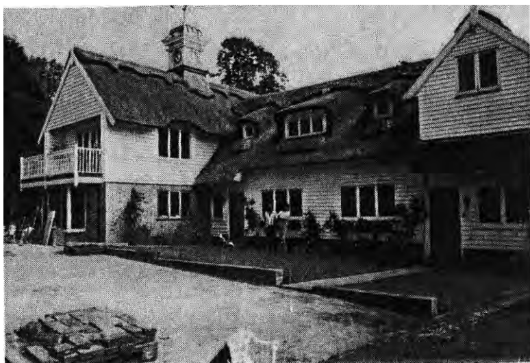
Photo 129 The converted stable block
