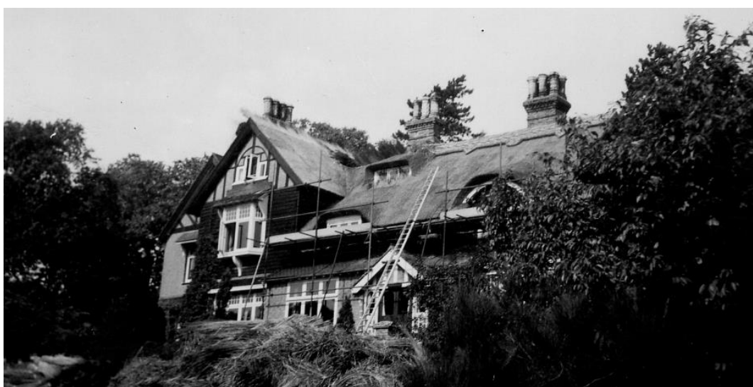
Photo 81 Thatching work on the house 1934
