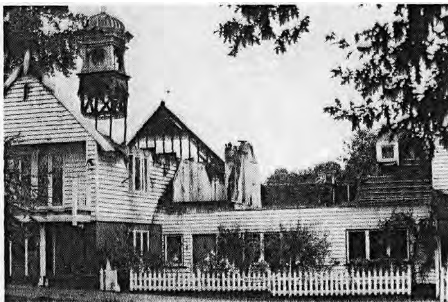
Photo 130 After the fire
